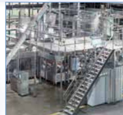
Supply air and exhaust air system on an aseptic filling machine
